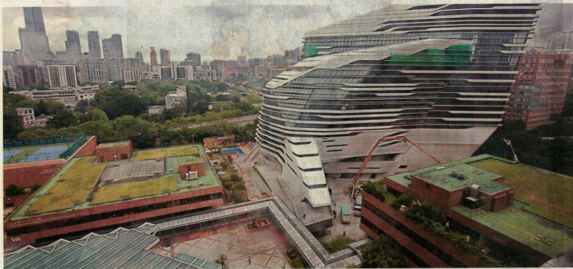
Grass is seen on rooftops at Polytechnic University, which has eight such features. Only five of them were submitted for Buildings Department approval. Photo: Edward Wong
